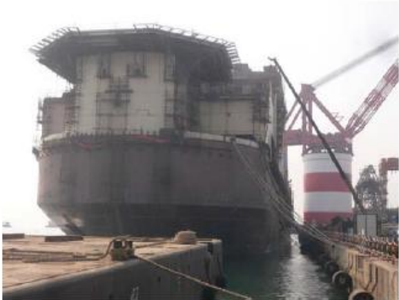
CastorOne at quayside
